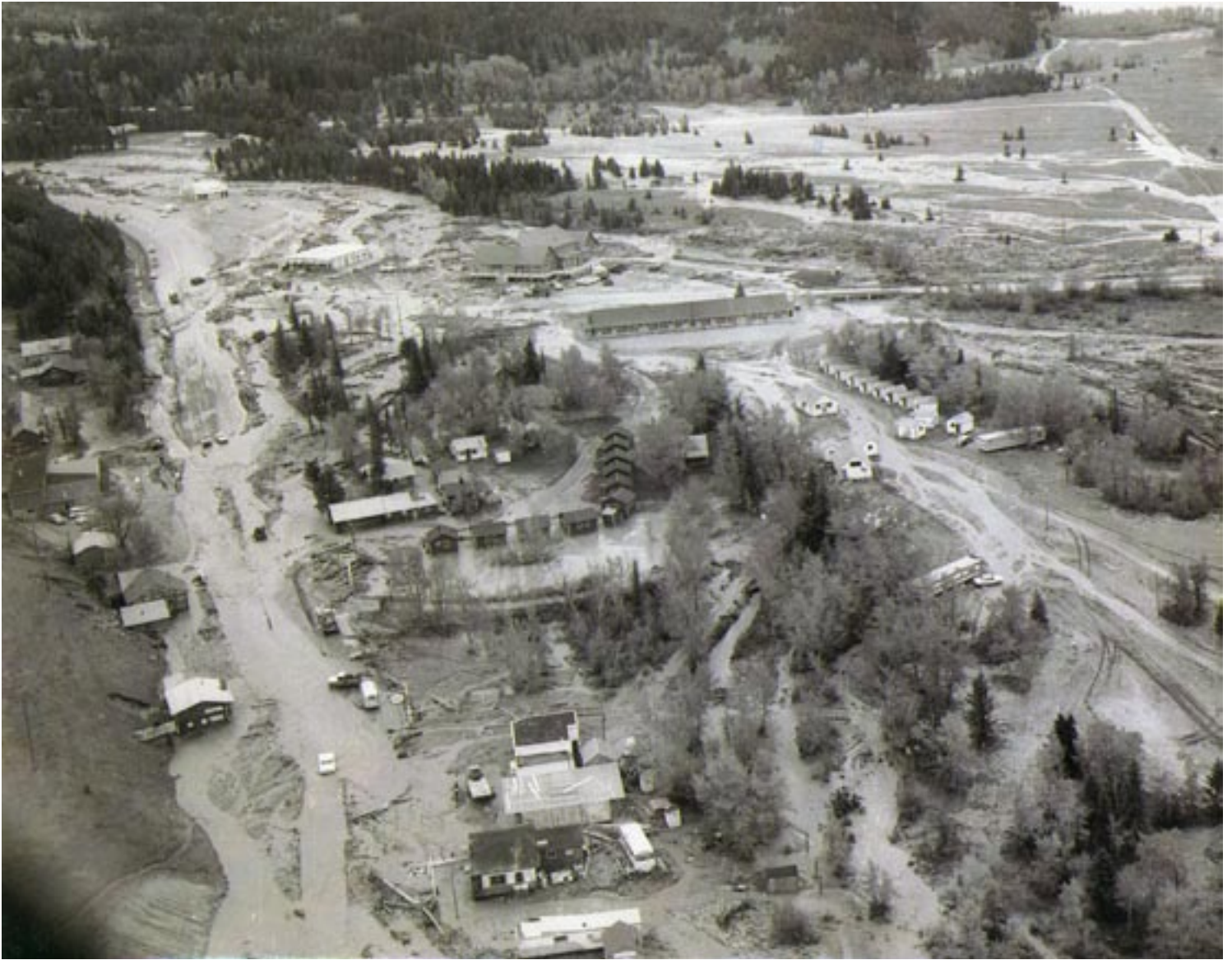
St. Mary Lodge and townsite during the 1964 flood. (Mel Ruder photo courtesy of Patsy Morton)
