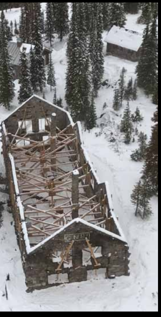
Sperry Chalet after the fire. Supports are already in place to support walls in preparation for reconstruction. (All Sperry photos courtesy of the National Park Service.)
